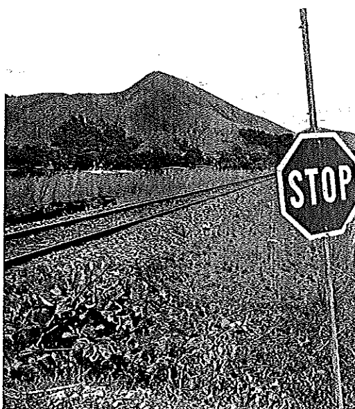
Significant investment is required to upgrade the railway network
