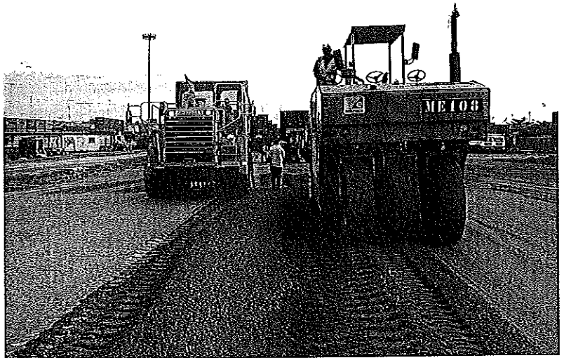
Existing roads are being rehabilitated and upgraded while new roads are also being built
